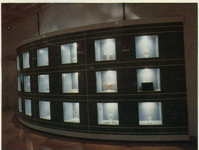
Glass pieces are housed in alcoves individually top lit with 50W 12V Myriad 40° beam downlighters.
