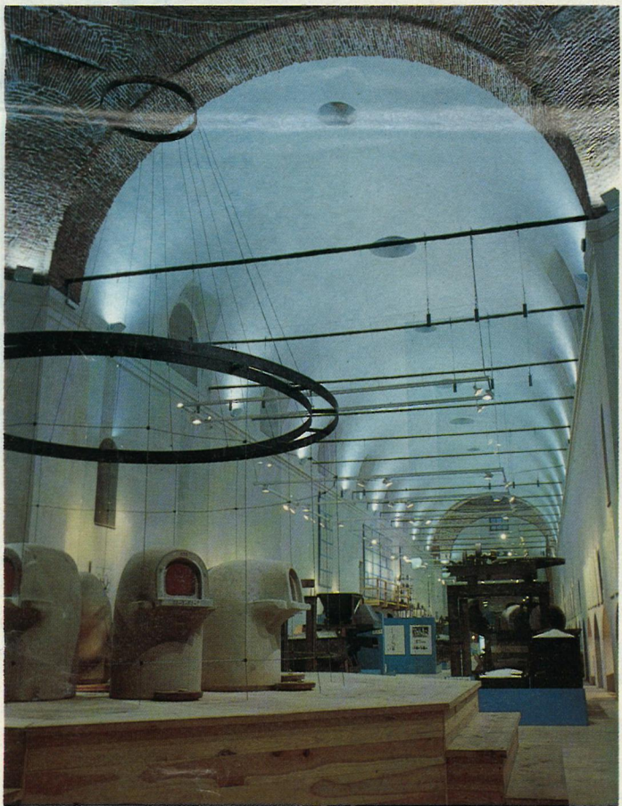
In this glass museum 70W metal halide uplighters recreate a 'daylight' wash that contrasts with the skeletal spotlight structure highlighting the exhibits.
