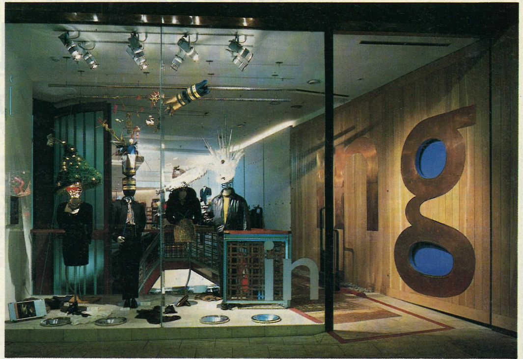
Metal halide uplighters with tungsten halogen spotlights on recessed Lytespan track in an ambient and accent combination.
